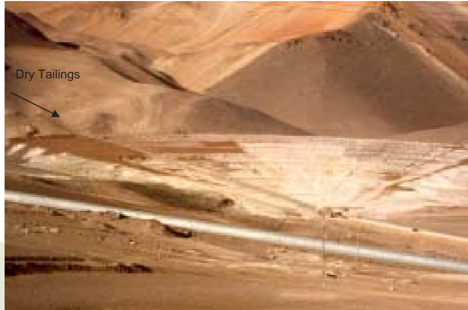
La Coipa Dry Stack Tailings Facility in the high Atacama Desert in Chile
